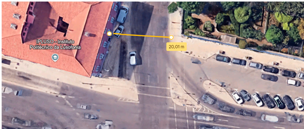
Figure 12. LOS scenario at 20m (GW at the window of the building and ED at the other side of the street in the sidewalk).
